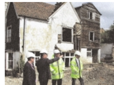
Perserving local heritage. Developing a new scheme for homeless people within the heart of historic Maidstone means building challenges as we preserve parts of the fifteenth-century Grade I listed building.
